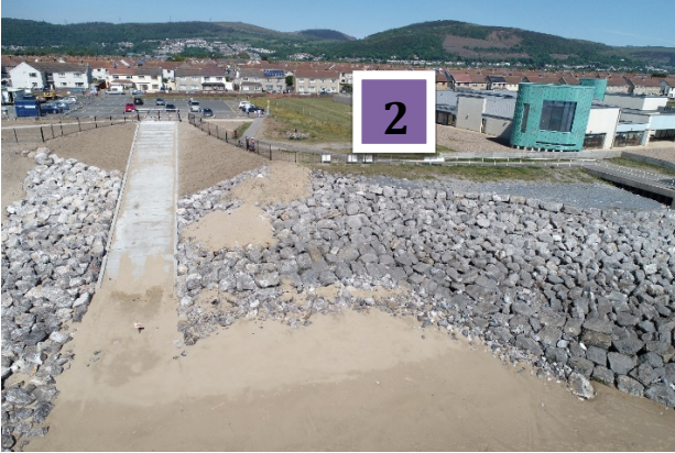
Figure 3 - Pedestrian access to the beach at East end of weldmesh fence
